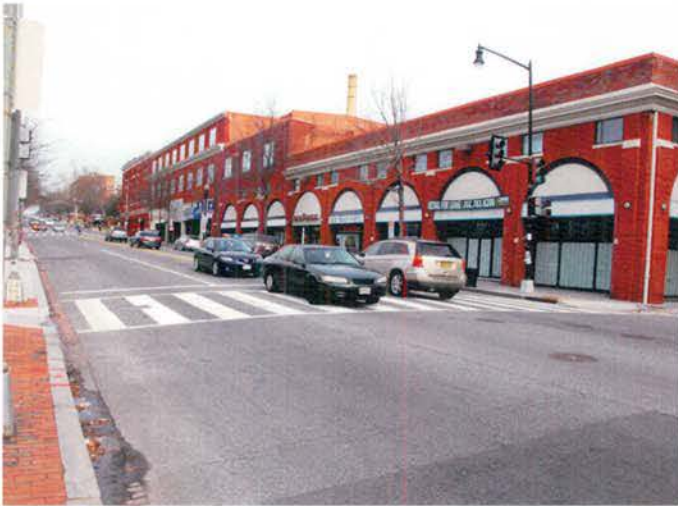
Photo 1-12: Existing view of Georgia Avenue and Bryant Street
